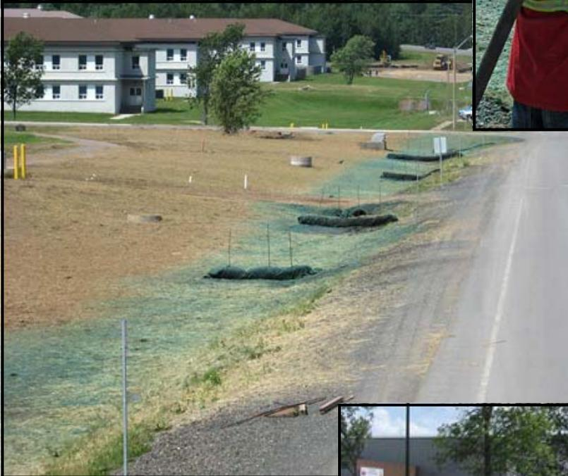
The contractor observed no problems or failure of the Flexterra-FGM, even though there was a rain event within one hour after the application. Stability was also maintained during the following 9 rainy days and there was no problem with sediment movement or brown water due to the addition of the Terra-Tube .
