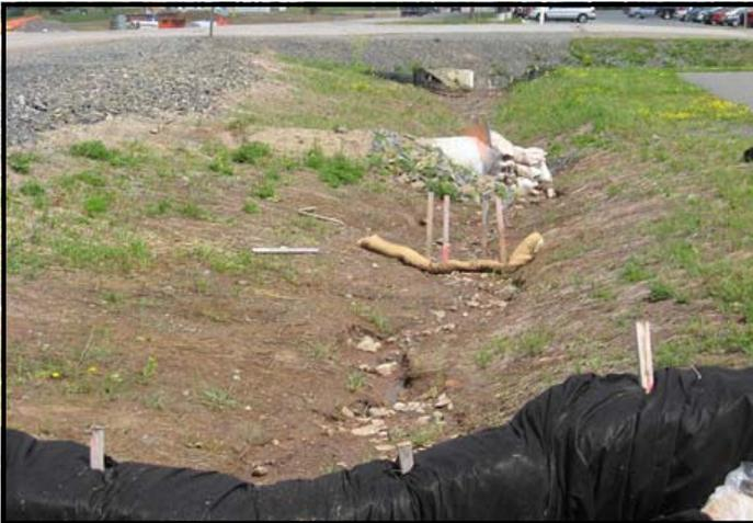
These photos show the condition of the site following the failure of the original Hydroseed application due to weather. Note the lack of turf growth, sediment movement and presence of brown water.
